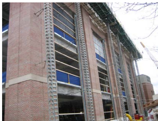
The east side of the building gets the finished brick exterior.
