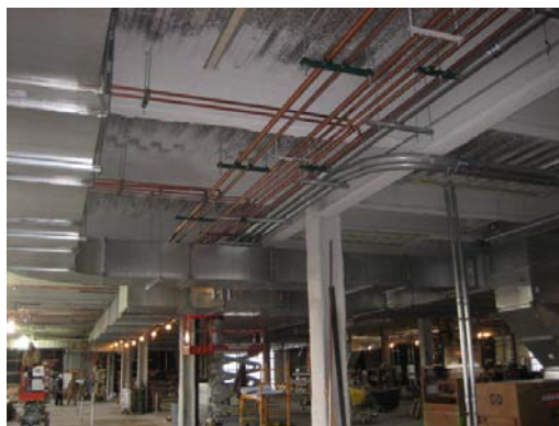
The plumbing is beginning to be installed.
